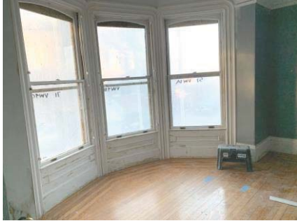
Kitchen- Demo done and framing done
